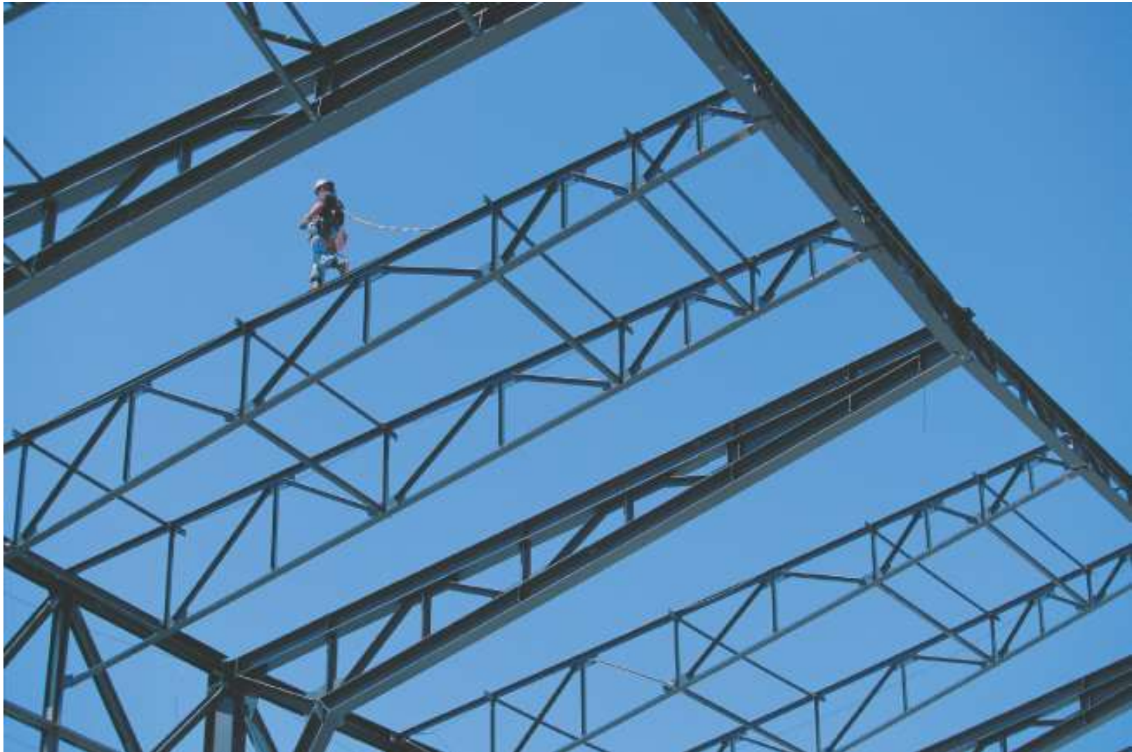
Roof trusses – Safeco Field in Seattle
