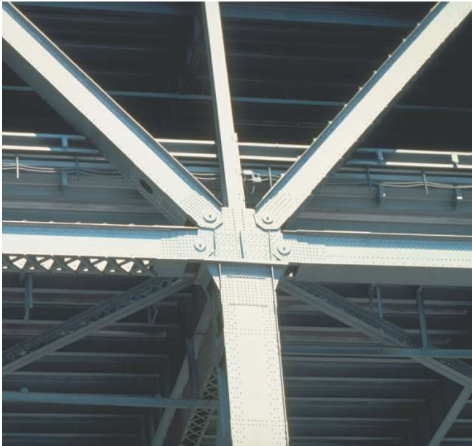
Photo 6.1 - Pin-jointed connection of the approach span to the San Francisco-Oakland Bay Bridge
